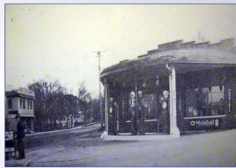
Hopkins and Walker Garage
