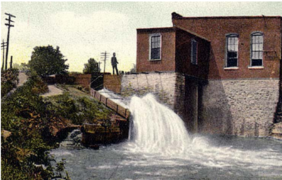
Dam and mill at White River outlet
